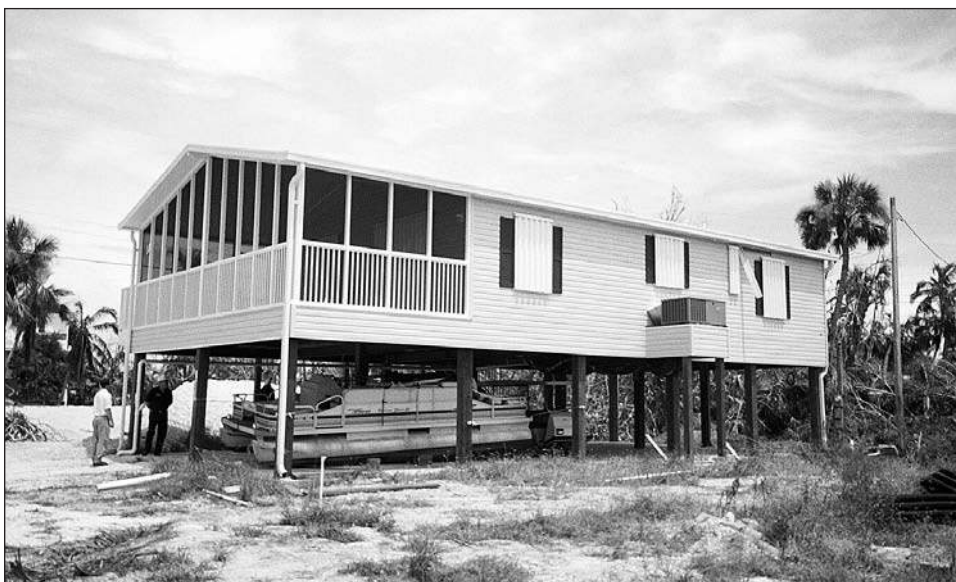
Figure 8-4. Manufactured home on a pile foundation.
