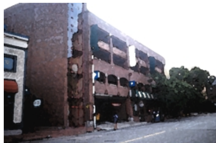
This parking garage, located in another community, contains characteristics such as retail uses on the ground floor, and an architecturally clad exterior that would be recommended as design considerations in the proposed Brazos Transit Center.
