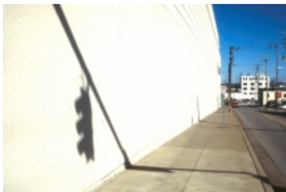
Building facades with no entrances, windows, or similar elements provide little visual interest, discourage pedestrian activity, and create "dead spaces" in the streetscape.
