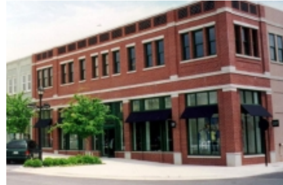
Awnings, pilasters, and vertically-oriented windows are used to create a series of bays that allow this new building to fit comfortably into a historic context.
