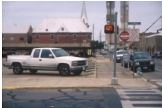
This corner parking lot, lacking any elements that define the street corner or screen the perimeter, was rated inappropriate by 75% of survey respondents who added that the scene looks "abandoned" and as if a "building is missing."
