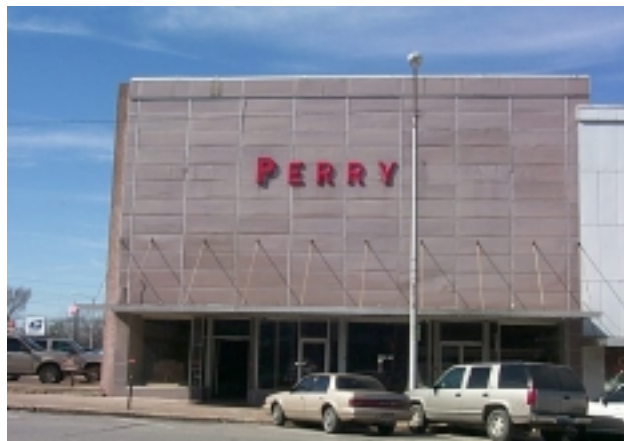
Inappropriate storefront alterations have diminished the character and historic integrity of some existing buildings. Fortunately, many such changes are reversible.
