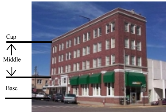
New buildings should employ a horizontal base and cap consistent with the tripartite building articulation historically found in Downtown Bryan. In this example, the base is the first floor of the building. In many examples found in Downtown Bryan, the base is articulated as a kick plate beneath front display windows.
