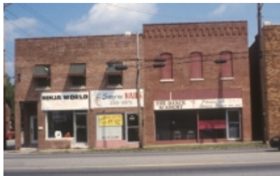
These facade-mounted signs lack visual cohesiveness, are inappropriately located on the facades, and utilize poor design and low quality materials. This sign image was the lowest rated in the survey, 96% inappropriate.
