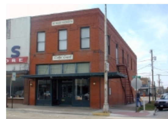
The facade of this building possesses many features appropriate for Downtown Bryan, including: vertically-oriented openings; well placed signage, transparency at the street level, clerestory windows and architecturally appropriate canopy.
