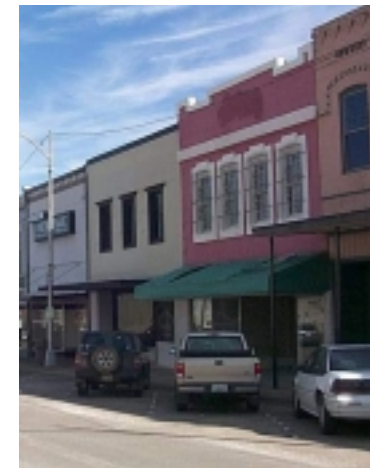
Characteristic of older commercial buildings, flat roofs with parapet walls should be the dominant roof form in Downtown Bryan.
