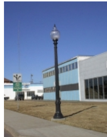
Typical 10-foot decorative light on Main Street between 28th and 29th
