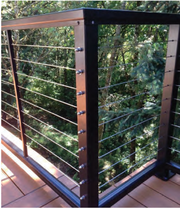
Cable rails/fencing painted black with stainless steel cables
