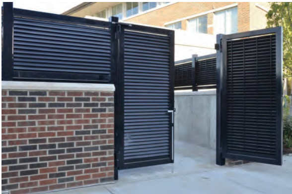
Screening - brick masonry, with louvered screens, painted black
