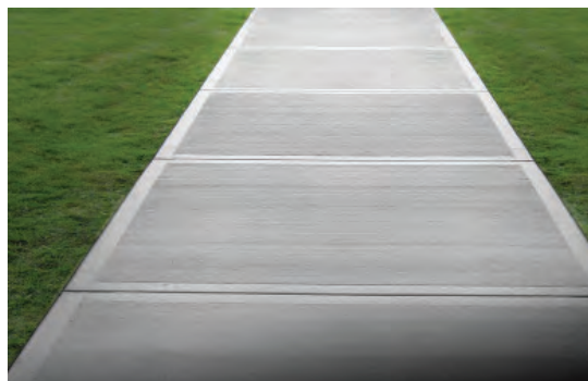
Concrete - Troweled edge with Broom Finish
